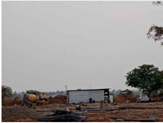
Beginning of construction activities on site
